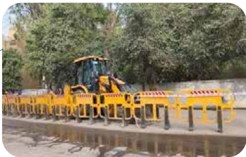
SEWER LAYING, MIRZAPUR
